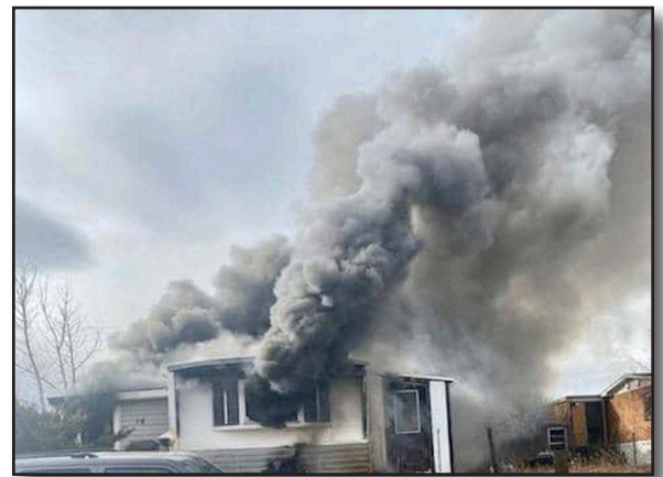
Figure 7-20 Reading Smoke - Velocity of smoke exits at different rates throughout the different openings
