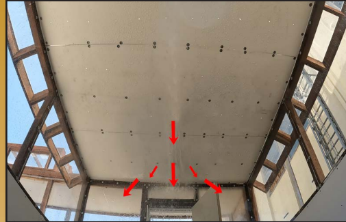
Improper - Shallow angle causes the stream to only make contact with backside of the compartment
