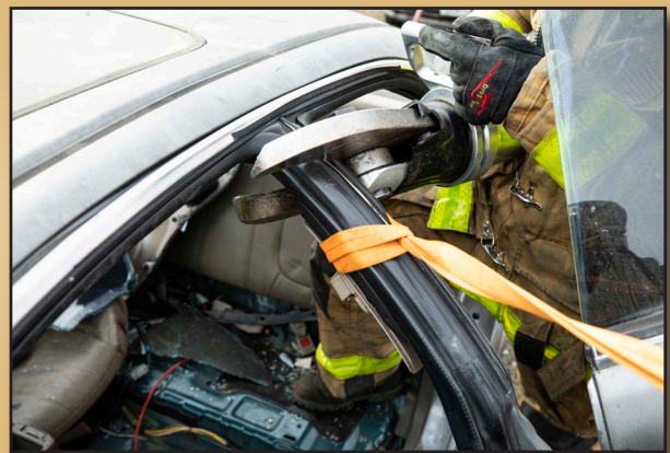
4. Cut the top B-Post as high as possible
