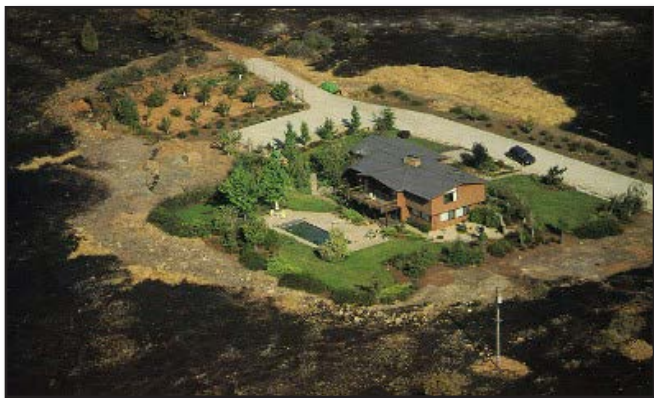
Figure 13-44 Threatened Defensible: 100' of defensible space, house can be used as a TRA, yard and road can be used as a safety zone.
