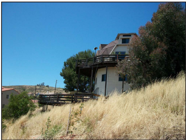
Figure 13-45 Threatened Non-Defensible: No clearing around structure, grass next to house and below wood deck, large trees close to house, house is midslope.
