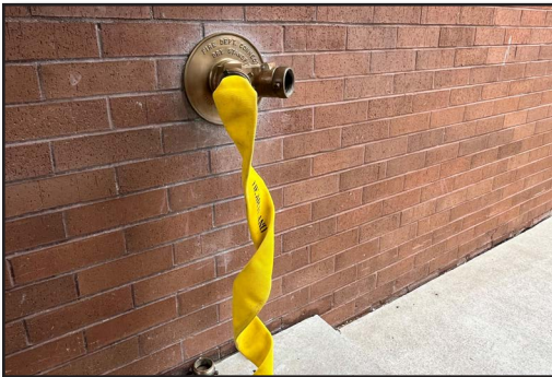
Figure 11-24 Twisting Hose to Connect to FDC
