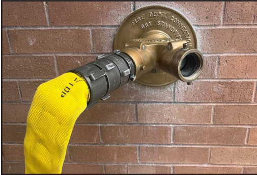
Figure 11-23 Double Female & Male Adaptor to FDC
