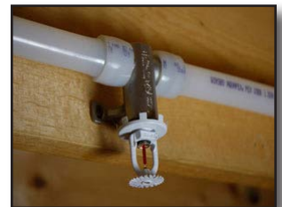
Figure 11-34 CPVC Sprinkler System Pipe
