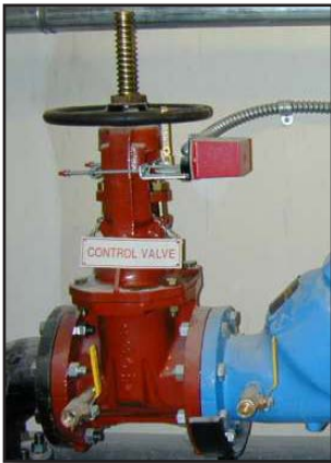
Figure 11-36 Outside Stem & Yoke Valve (OS&Y)
