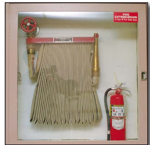
Figure 11-18 Class II Standpipe System
