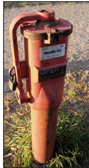
Figure 11-37 Post Indicator Valve (left), Wall Post Indicator Valve (top right), Indicating Butterfly Valve (bottom right)
