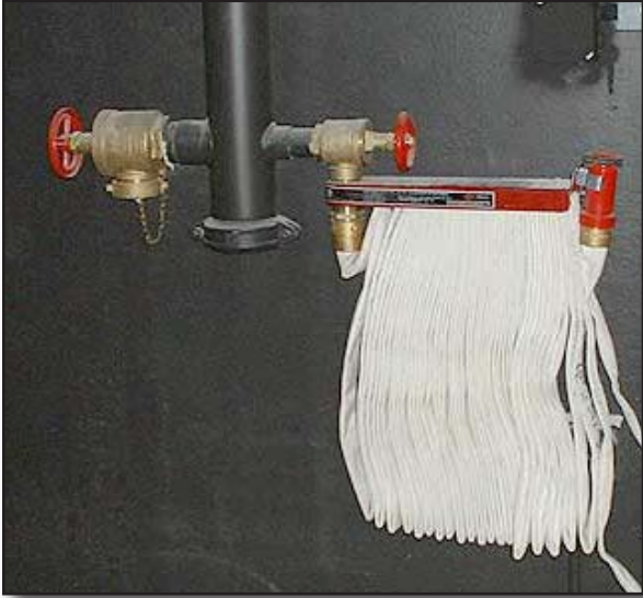
Figure 11-19 Class III Standpipe System
