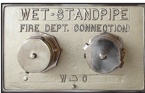
Figure 11-20 Automatic-Wet Standpipe Connection
