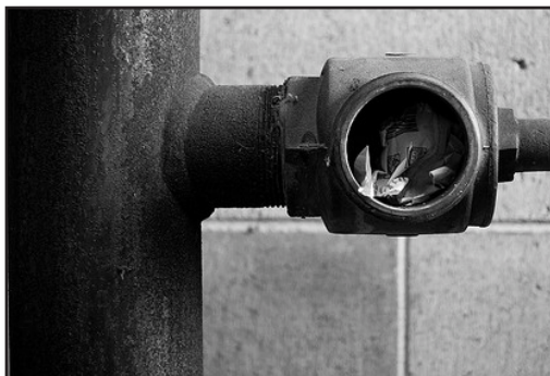
Figure 11-25 Standpipe Obstruction
