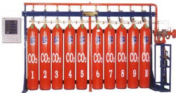
Figure 11-49 Carbon Dioxide System Storage Tanks
