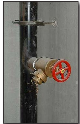
Figure 11-17 Class I Standpipe System
