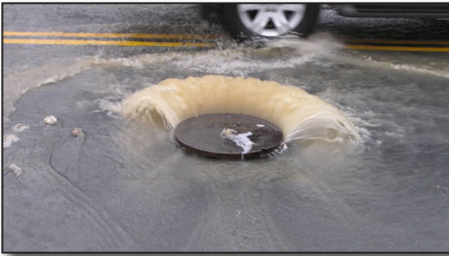
Figure 37-17 During periods of significant rainfall, storm drain systems often become overwhelmed. This results in a buildup of water pressure that is powerful enough to dislodge and move manhole covers (picture on left). When a manhole cover has been dislodged and water begins to recede, a drain path is created. These situations are extremely dangerous for rescuers and may not be as visible from the surface or as obvious as the picture on the right.
