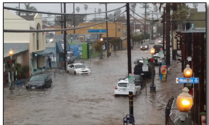
Figure 37-8 Seasonal flooding on the streets of Ocean Beach due to heavy rainfall.
