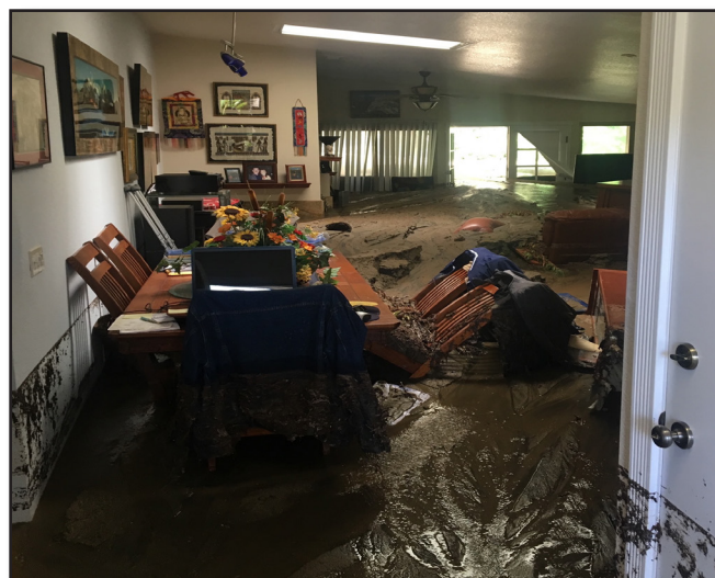
Figure 37-6 A broken water main in the hillside above this home in 20's district caused a significant mud flow that filled the entire home in a matter of minutes. Fortunately, the homeowner was able to escape unharmed despite the structure being a total loss. 2018.
