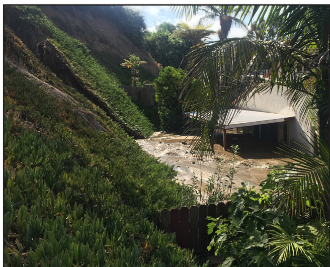
Figure 37-6 A broken water main in the hillside above this home in 20's district caused a significant mud flow that filled the entire home in a matter of minutes. Fortunately, the homeowner was able to escape unharmed despite the structure being a total loss. 2018.
