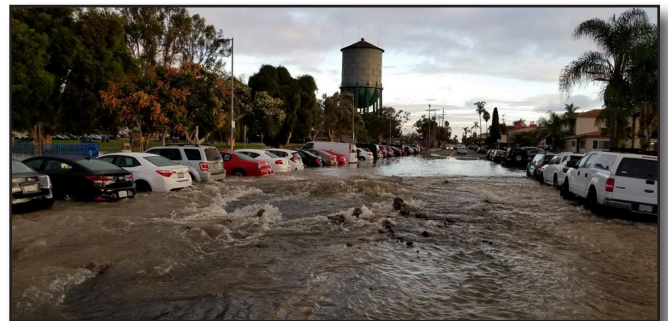
Figure 37-7 A broken water main flooded the streets of North Park caused an out of season swiftwater environment.
