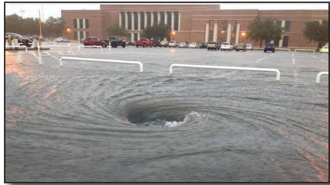
Figure 37-17 During periods of significant rainfall, storm drain systems often become overwhelmed. This results in a buildup of water pressure that is powerful enough to dislodge and move manhole covers (picture on left). When a manhole cover has been dislodged and water begins to recede, a drain path is created. These situations are extremely dangerous for rescuers and may not be as visible from the surface or as obvious as the picture on the right.
