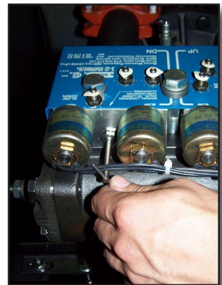
Figure 32-24 Typical hydraulic elevator bleeder valve control
