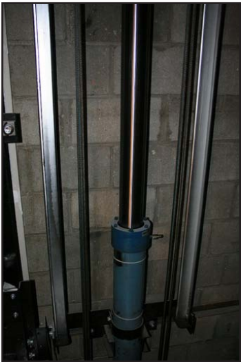
Figure 32-6 Hydraulic Elevator Ram
