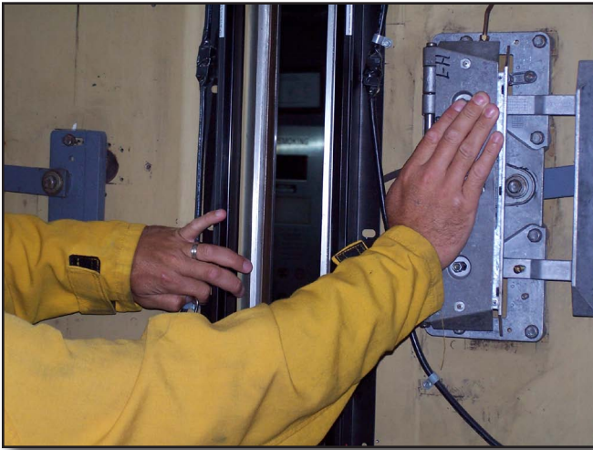
Figure 32-23 By pressing on the elevator car door clutch assembly you can easily open the car/cab doors
