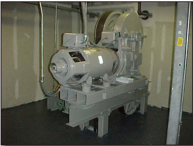
Figure 32-14 Traction Electric Hoisting Machine/Motor
