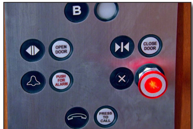
Figure 32-17 When activated, the Emergency Stop Button (red pull switch) will not allow Phase I operations and resetting the power to restore the elevator to a working condition.
