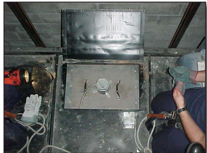
Figure 32-11 Elevator Car Roof Escape Hatch (top view)
