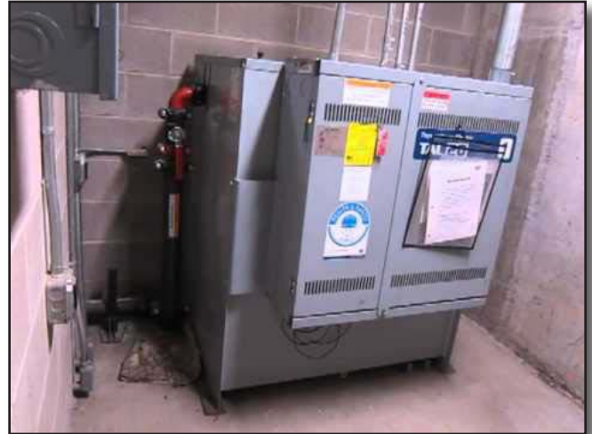
Figure 32-15 Hydraulic Elevator Machine/Pump
