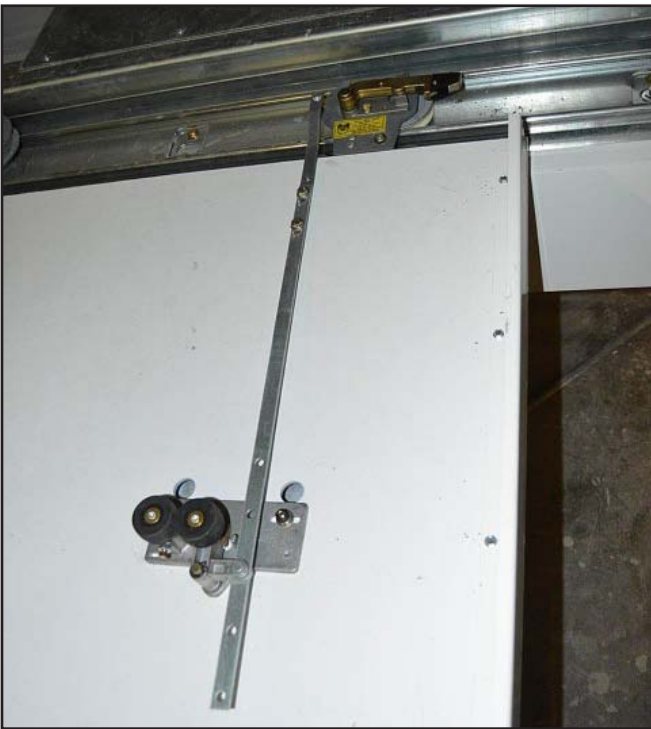
Figure 32-3 Interlock & Pick-up Rollers
