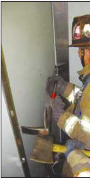
Figure 32-22 The use of a forcible entry tool can often provide enough force to override/break the interlock and allow the doors to open while causing minimal damage
