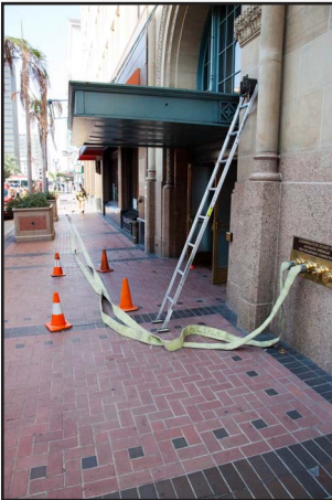
Figure 31-53 Connect a minimum of two supply lines to the FDC and set up two engine companies to pump in series.
