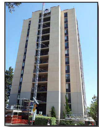
Figure 31-6 Smoke Tower with outside vestibule
