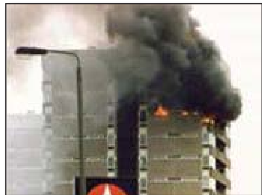
Figure 31-15 Un-compartmentalized fires should be attacked using 2 1/2” hose
