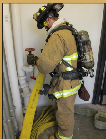
Connect to the standpipe one floor below the fire floor and flake the remaining hose down that floor's hallway
