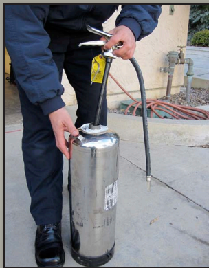
Remove nozzle & pick-up tube assembly
