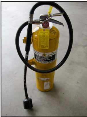
Figure 10-16 Stored pressure Class D extinguisher
