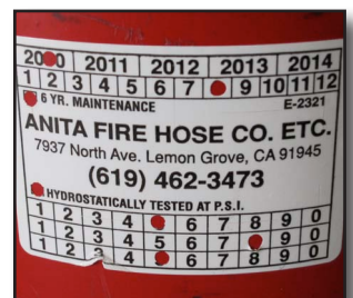
Figure 10-18 Extinguisher service tag
