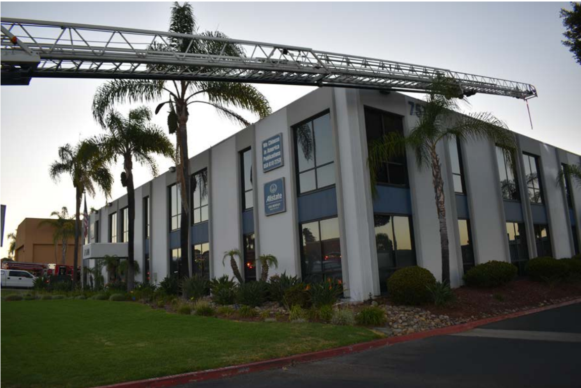
Photo No. 4: Aerial ladder placement at Alpha – Delta Corner
