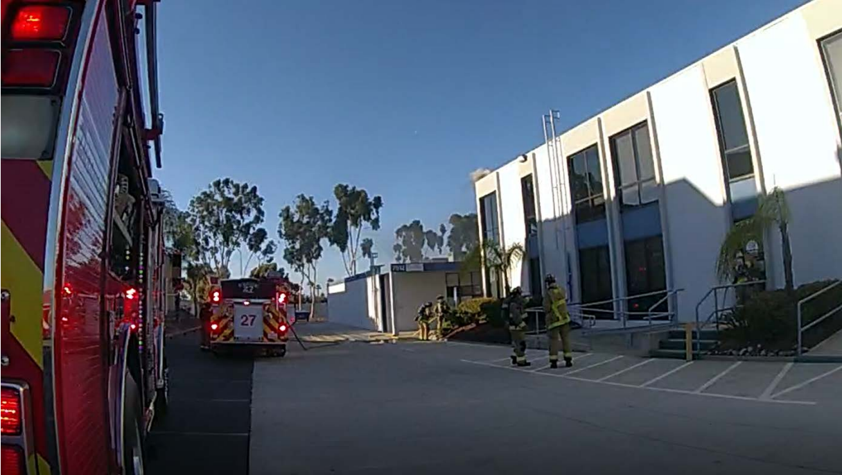
Photo No. 15: View of forcible entry operation at entry door and suppression efforts at B-C corner
