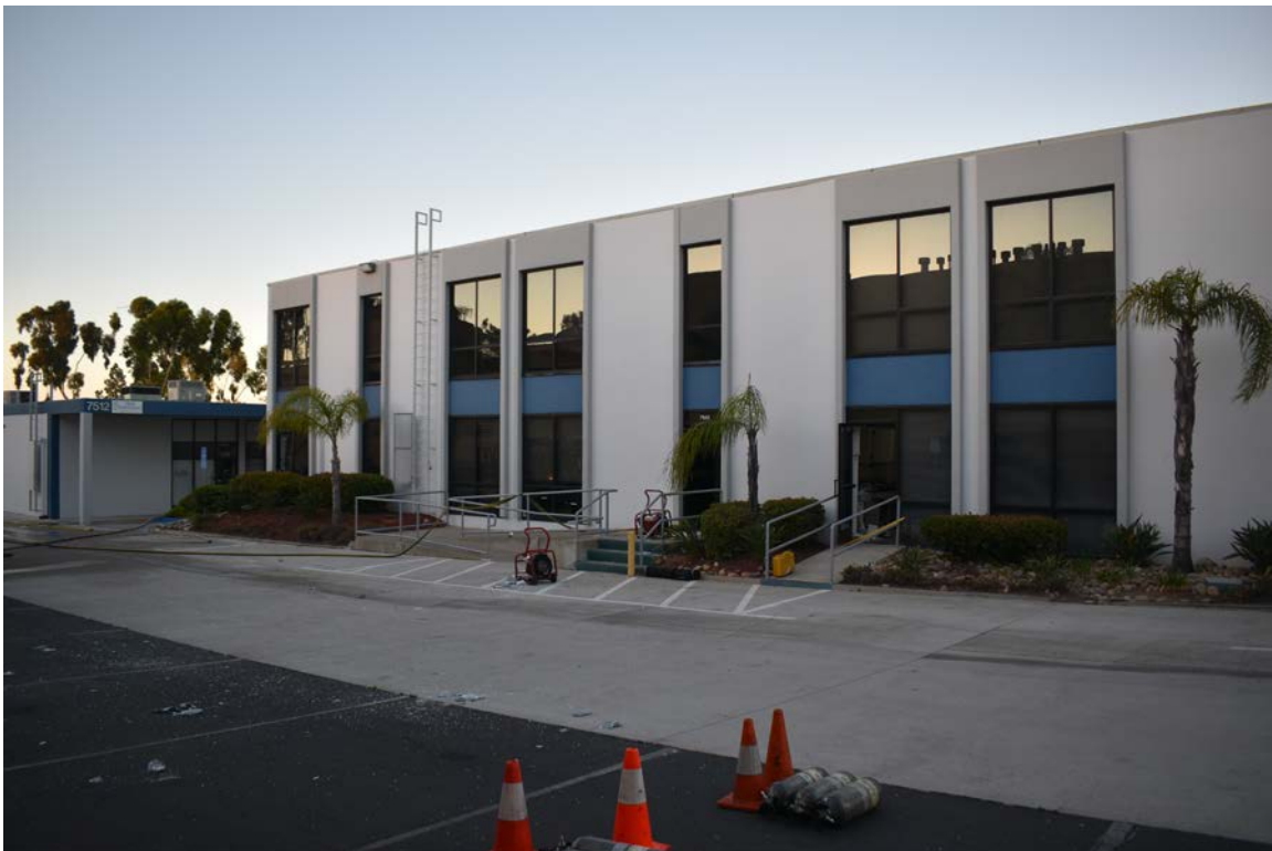
Photo No. 2: Bravo side of structure. Location of event.
