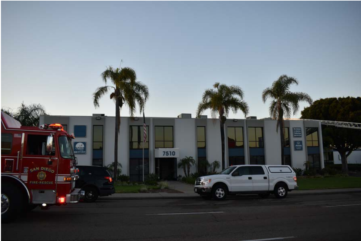
Photo No. 1: Alpha side of two story commercial structure with center courtyard.
