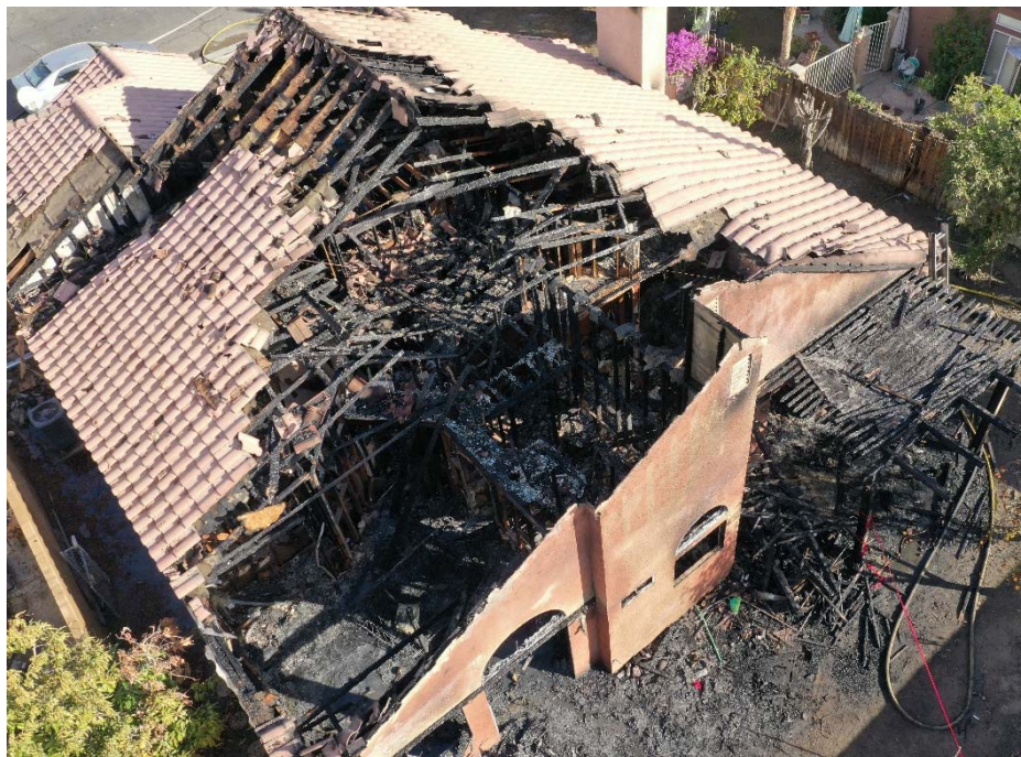
Photo 7: Aerial view of C/D corner of the structure
