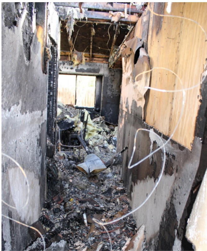
Photo 3: View from master hallway looking towards C/D corner
