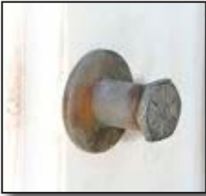
Figure 25-3 Nader Pin
