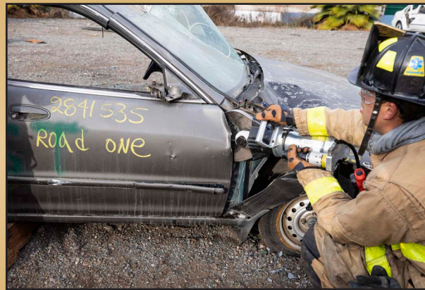
4. Place your cutter tool in the newly created space and cut both door hinges
