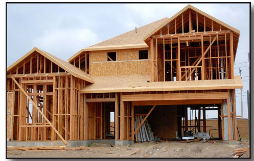
Figure 8-50 Type V Construction
