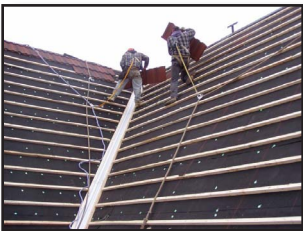
Figure 8-36 Batten Grid System for Metal Roof
