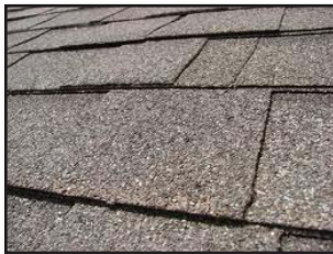
Figure 8-29 Asphalt Composition Shingle
