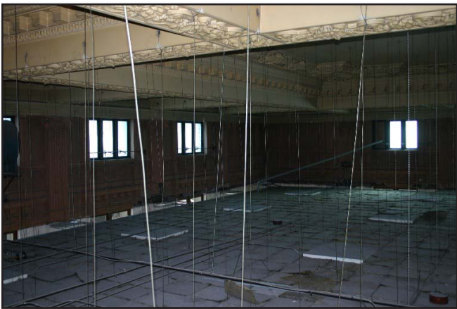
Figure 8-44 The plenum, or space above a suspended ceiling
