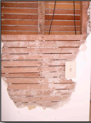
Figure 8-25 Lathe & Plaster construction
