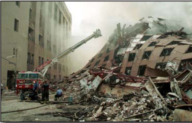
Figure 8-1 Building Collapse - FDNY
