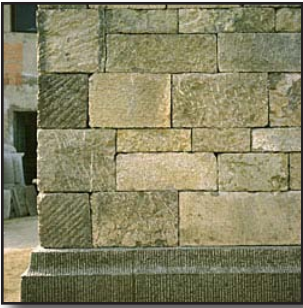
Figure 8-5 Solid Stone Construction
