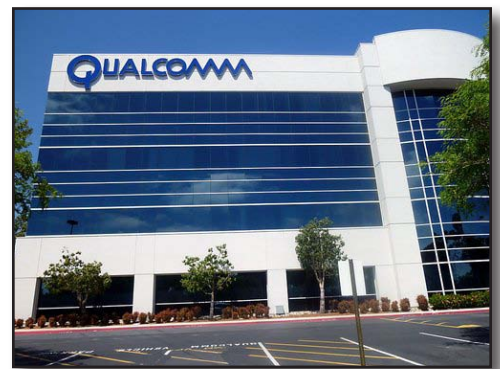
Figure 8-45 Type I Construction
