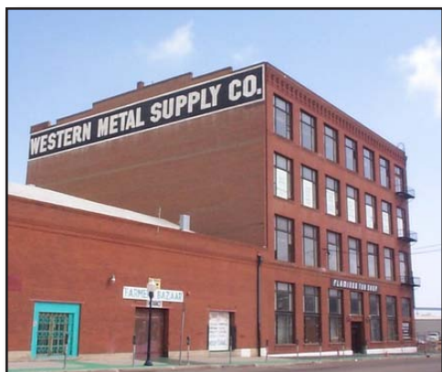
Figure 8-47 Type III Construction
