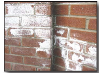
Figure 8-7 Efflorescence
