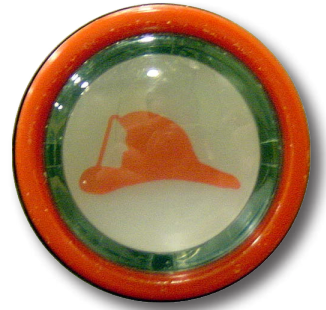
Figure 31-48 When the fire helmet pictograph is flashing, do not use elevator.
