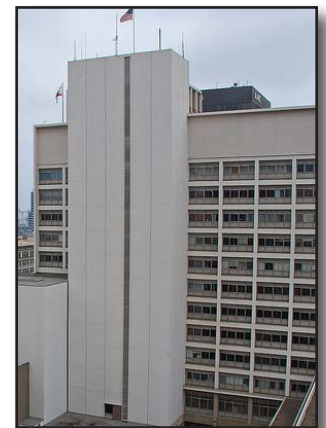
Figure 31-9 San Diego City Hall - Existing High-Rise
