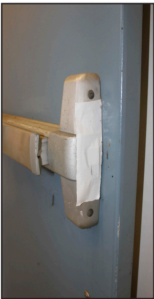
Figure 31-34 Duct tape placed over the door latch allows the door to close for stairwell pressurization but not lock you out
