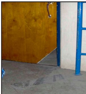
Figure 31-20 Notching the bottom corner of the door will prevent smoke from entering the stairwell during fire attack
