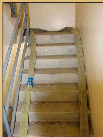
Leaving the nozzle in place, flake the first 50' to 75' of hose up the stairwell above the fire floor if conditions permit
