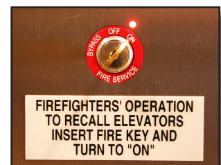
Figure 31-46 Phase I elevator operation occurs from the elevator lobby and is used to recall the elevator to the main floor
