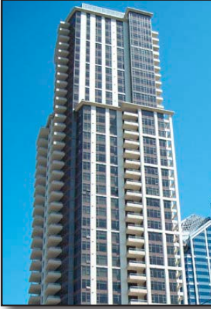
Figure 31-10 San Diego's "Electra" Residential Life Safety High-Rise, 2007
