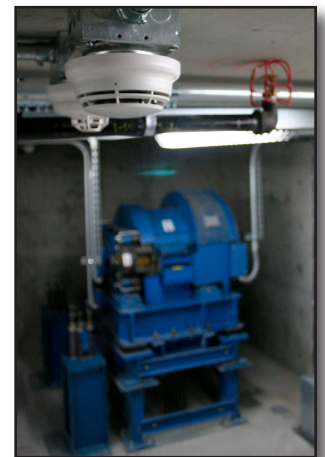
Figure 31-49 An activated Fire Alarm Initiating Device (FAID) inside of the elevator machine room will send the elevators into Automatic Phase I Recall - Do Not Use!
