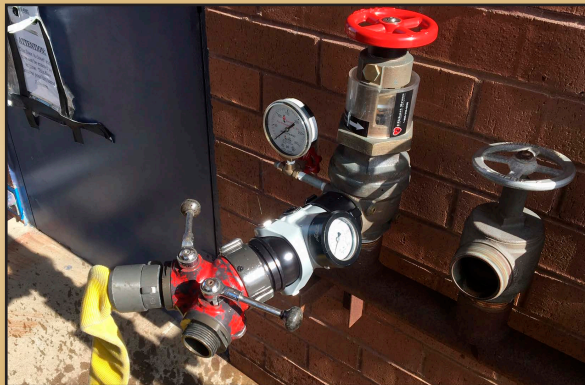
Attach the in-line pressure gauge, gated wye, and hosepack A to the standpipe outlet, one floor below the fire floor, spanner tight
