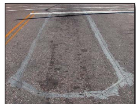
Figure 21-46 Magnetic sensor imbedded in the asphalt opens security gates from the inside.
