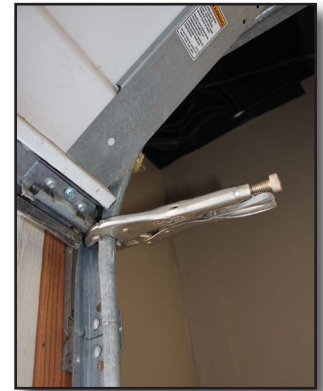
Figure 21-38 Channel Locks used to clamp sectional door open
