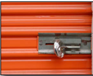
Figure 21-35 Slide Bolt & Lock Mechanism
