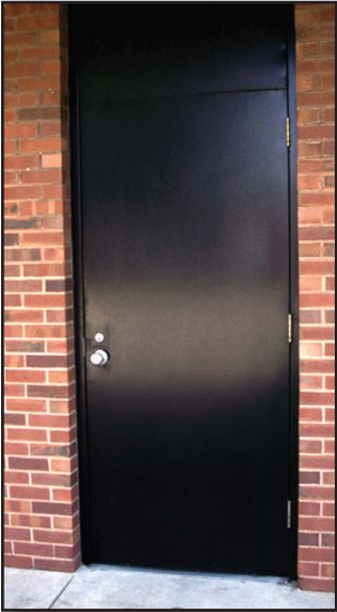
Figure 21-13 Outward Swinging Door
