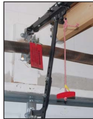
Figure 21-39 Manual disengage lever/cord for electrically operated doors
