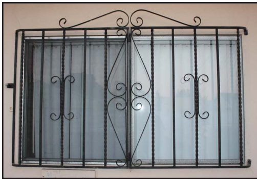
Figure 21-59 Security bars mounted on the outside of the window
