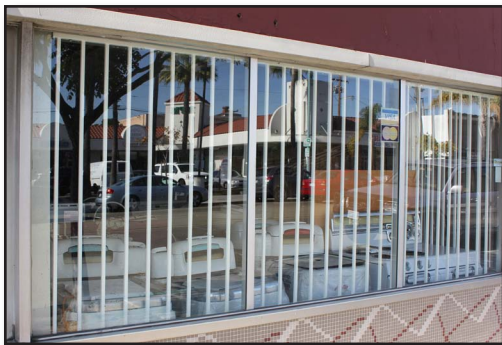
Figure 21-60 Security bars mounted on the inside of the window
