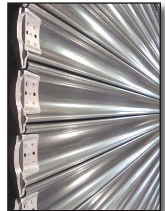
Figure 21-42 Interlocking slats may be riveted together on the ends which may prevent them from being pulled out
