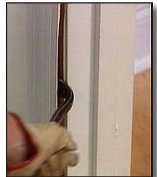
Figure 21-7 Removing the stop from the door jamb
