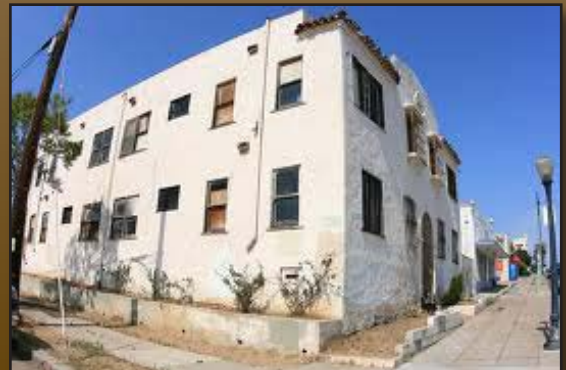
Abandoned Apartment Bldg
