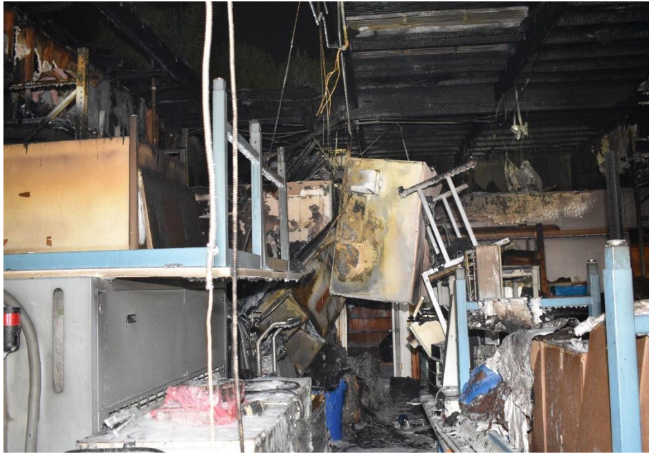
Interior, noted A/C unit (center, suspended)
